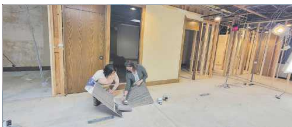
Remodeling is beginning in the old US Bank building
